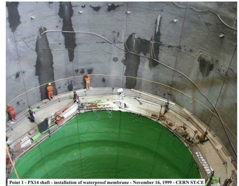
Point 1 - PX14 shaft - installation of waterproof membrane - November 16, 1999 - CERN ST-CE
